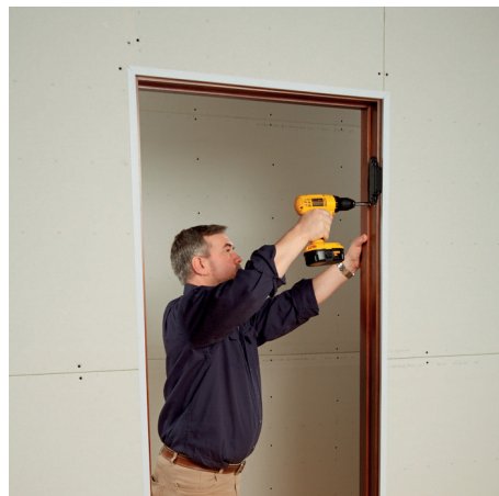
⚠️ MOUNT CONCEALED HINGES TO JAMB FIRST USING SUPPLIED SCREWS.
