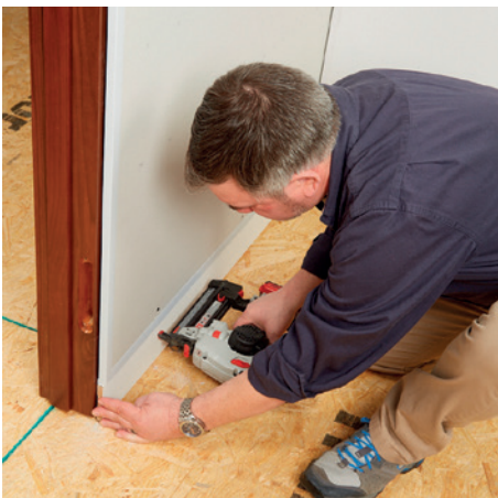
Trim remaining drywall and install baseboard.
