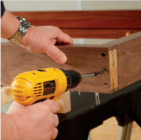
Assemble and install jamb before hanging drywall.
