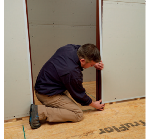
Finish drywall edges with U-bead, J-bead or similar drywall trim.
