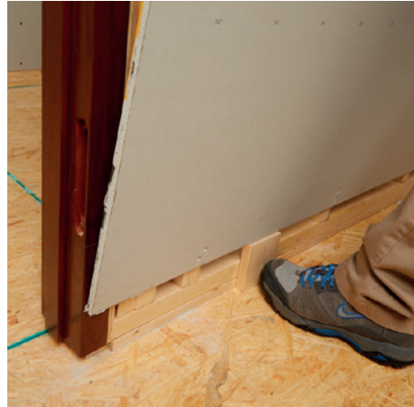
Lift drywall to baseboard height using a block for support. Overlap jamb with drywall to create the desired amount of reveal.
