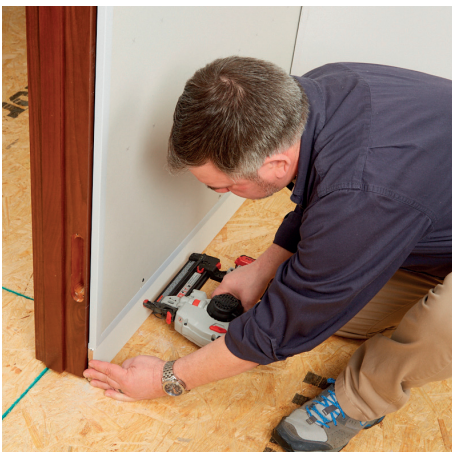
Trim remaining drywall and install baseboard.
