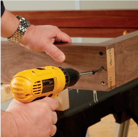
Assemble and install jamb before hanging drywall.
