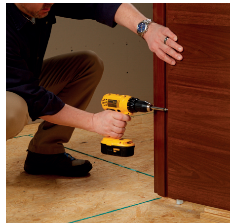
Align door with hinges and mount with provided screws. Adjust hinges if necessary and attach cover plate.
