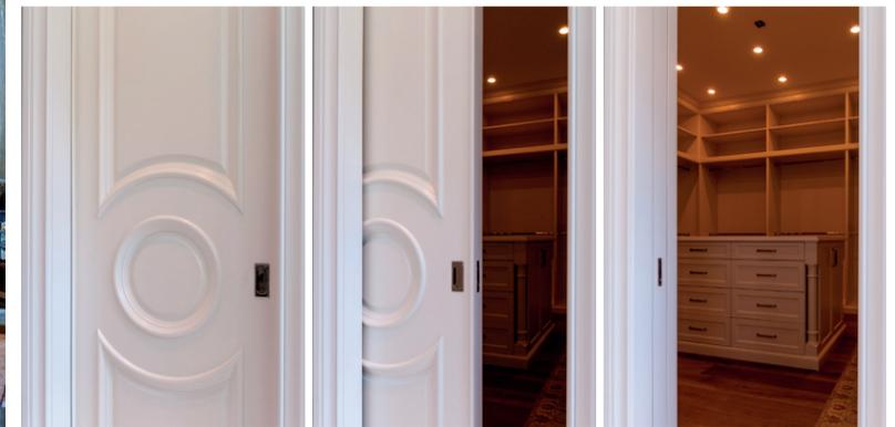
The clever addition of trim applied to the sides of pocket doors allows highly sculpted big bolection moulding to be used. The trim covers the pocket opening when doors are open or closed.
